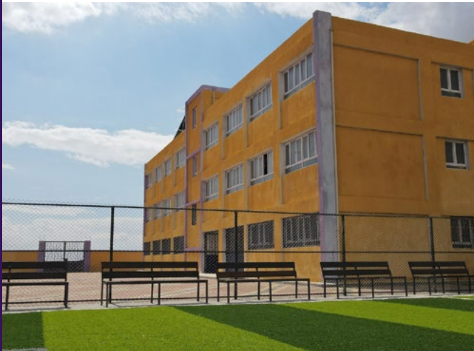
A view of Al-Zohoor school from the football field.
