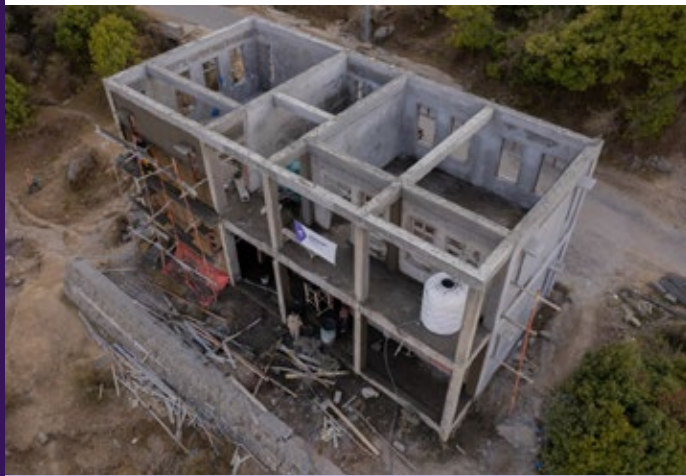
Chitratopi school under construction.
