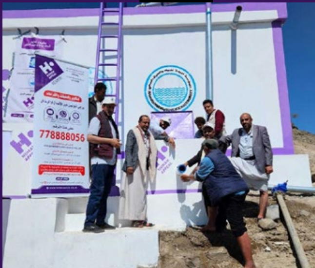
The completed Al Qefr water tank.
